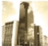
CERRITO OFFICE TOWER
